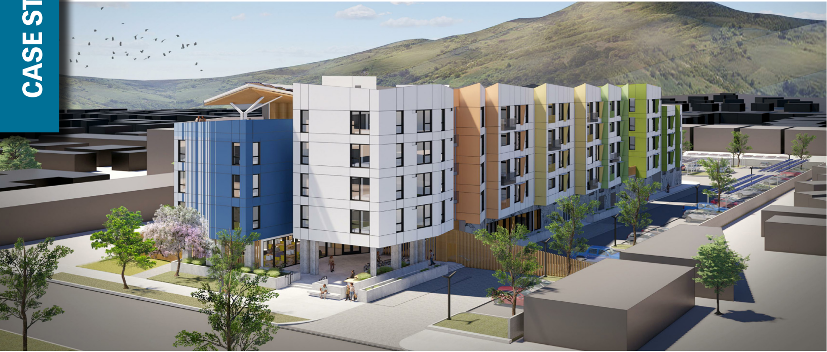
THE MAGNOLIAS, AFFORDABLE MODULAR HOUSING, MORGAN HILL, CALIFORNIA
